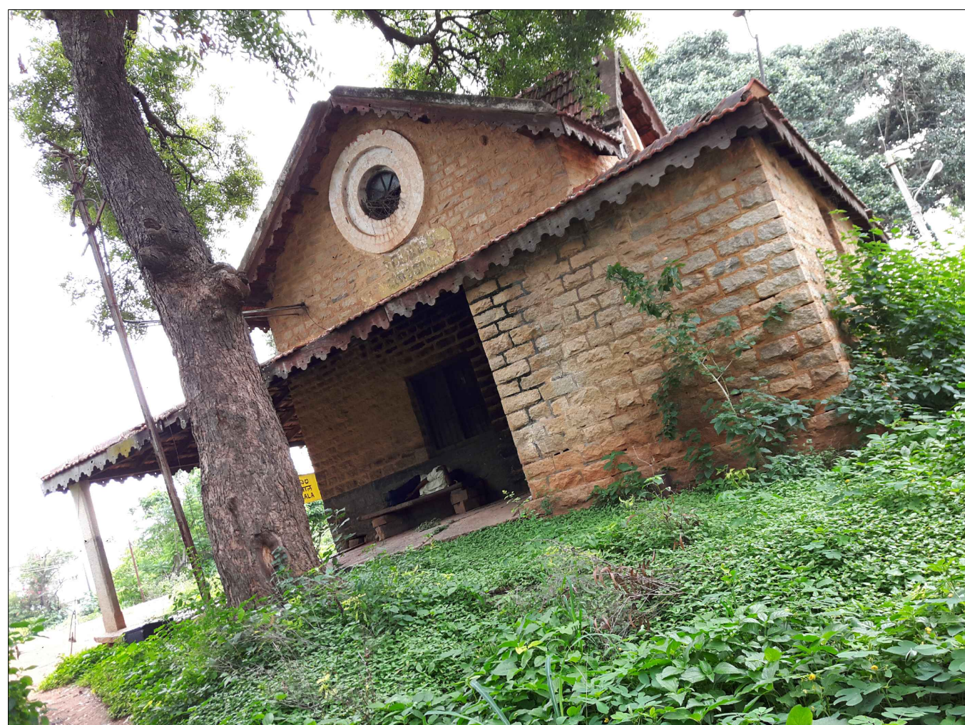
(Source: Photo Taken by Ar. Sharan Desai)
